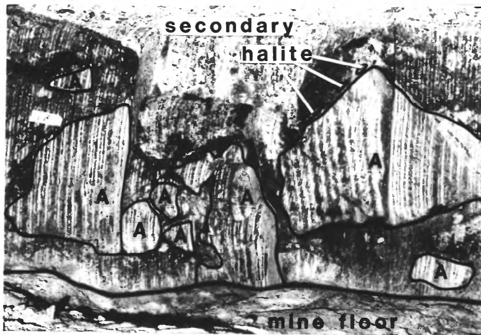
Figure 19.--Left side of exposed breccia pipe at end of 16-L drift showing numerous anhydrite blocks and matrix of clay and halite and anhydrite fragments. A=anhydrite.
